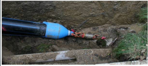
12" QUICKCONNECT PULL HEAD W/ HDPE
